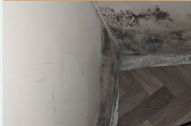
Photos from one month after repairs
